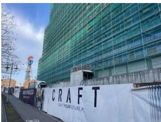
View of the office building from the south side
