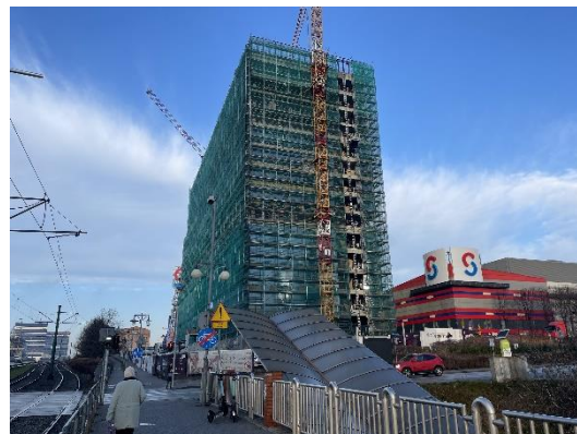
View of the office building from the east side
