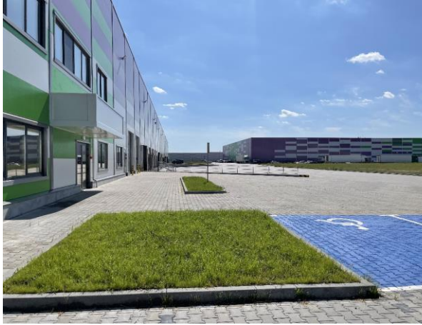
View of the Logistics complex
