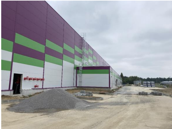
BTS Stokrotka – western facade
