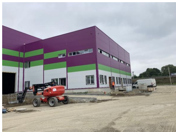
BTS Stokrotka – northern facade
