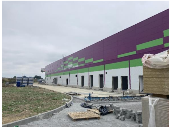
BTS Stokrotka – western facade
