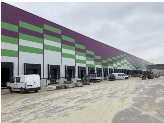
BTS Stokrotka – northern facade
